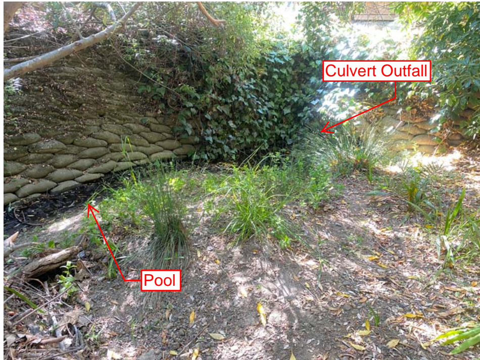
Photo 1. View of culvert outfall and stacked concrete bags below homes on Jeffrey Avenue with a small narrow pool of water approximately 4 inches deep.
