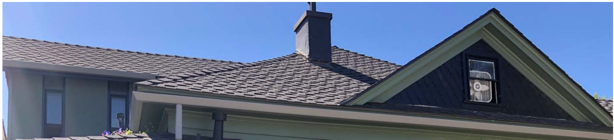
Above: later pushout, in part possibly dating before 1965, with modern bay window, north façade. Below: The north façade pediment gable, with original diamond and scalloped wall shingle, altered by the insertion of a later window to make the attic habitable. The chimney is also a later addition.
