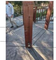
PROVIDE AND INSTALL NEW GALVANIZED RIGID STEEL CONDUIT FROM JB1 TO JB3, SEE DETAIL 3 ON THIS SHEET, PROVIDE 2-HOLE PIPE STRAPS EVERY 36' ON NEW CONDUIT, PAINT CONDUIT TO MATCH EXISTING GAZEBO.
