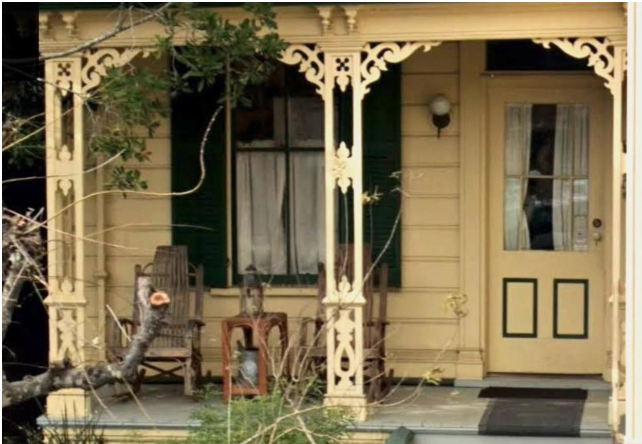
The Squibb House pierced columns, with elaborate fretwork inserts apparently never present in the pierced columns of the Bianchini and Music Houses
