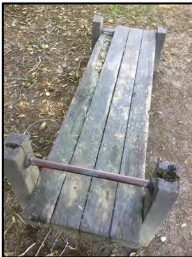
Figure 9a. Adult fitness equipment missing a backboard
