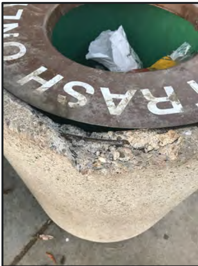
Figure 4d. Chipped trash can located near park entrance
