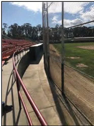
Figure 24e. Potentially dangerous railing for children
