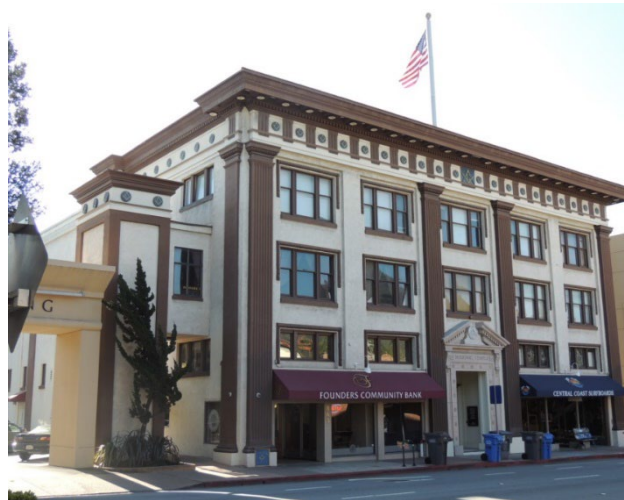
Masonic Temple, 856 Marsh Street, built 1913. Source: Historic Resources Group (2013).
