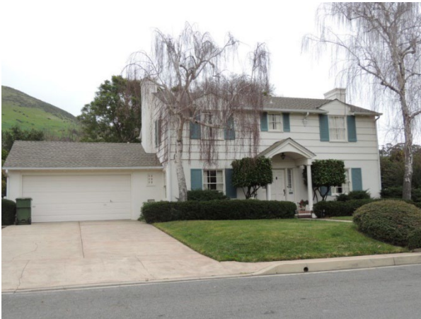
1727 Corralitos Avenue, built c.1940. Source: Historic Resources Group (2013).
