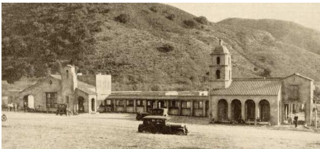
Milestone Mo-tel, 2223 Monterey Street, built 1925. Source: Huntington Library, San Marino.
