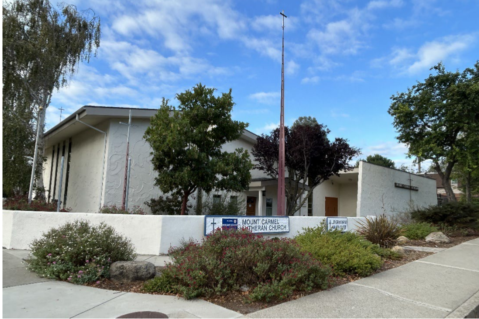
George Hasslein, Mount Carmel Lutheran Church, 1701 Fredericks Street, built 1958. Source: Page & Turnbull (2025).
