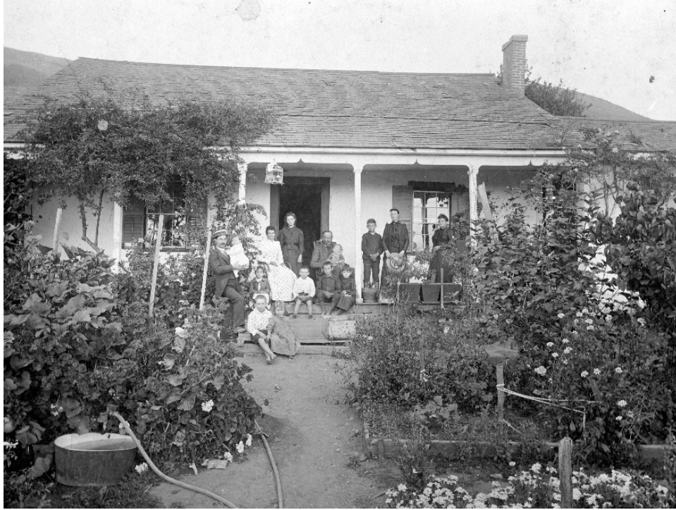
Andrews Adobe, 1451 Andrews Street, built c. 1830. Designated as a San Luis Obispo Historic Landmark. Source: San Luis Obispo County Regional Photograph Collection, Cal Poly Special Collections (c. 1890-1906).
