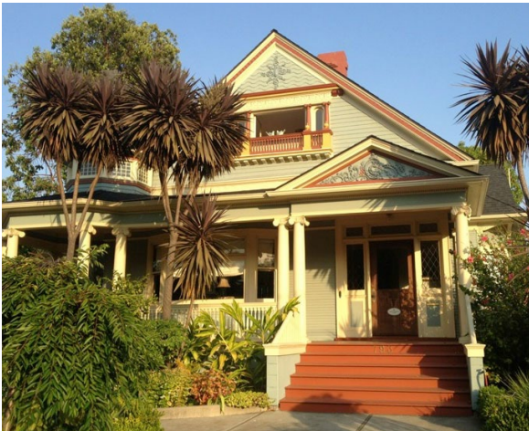
Crocker House, 793 Buchon Street, built 1901-1902. Source: City of San Luis Obispo.
