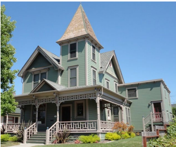
McManus House, 639 Pismo Street, built 1901. Source: City of San Luis Obispo.
