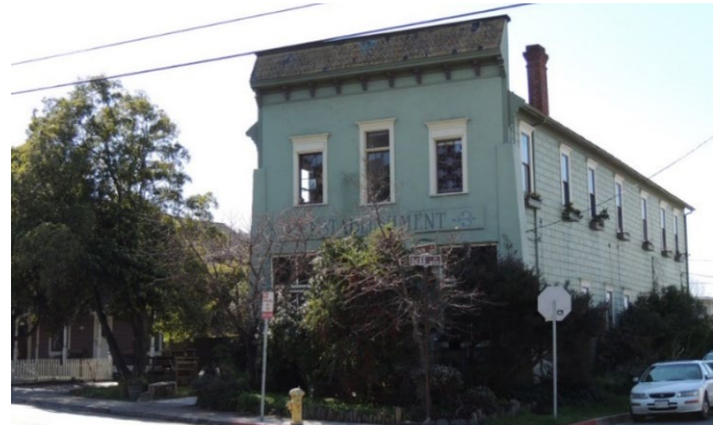
Call Hotel, 1703 Santa Barbara Street, built 1895. Designated as a San Luis Obispo Historic Landmark. Source: Historic Resources Group (2013).
