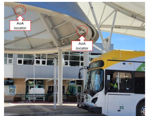
Image – AoA locators installed at Solano County Transit (SolTrans).
