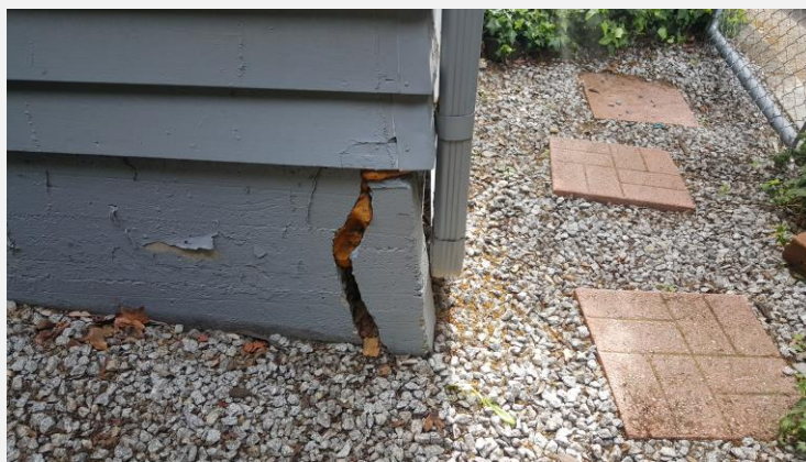
Figure 3: Foundation Cracking at 1016 Walnut St., the “Blue House”
