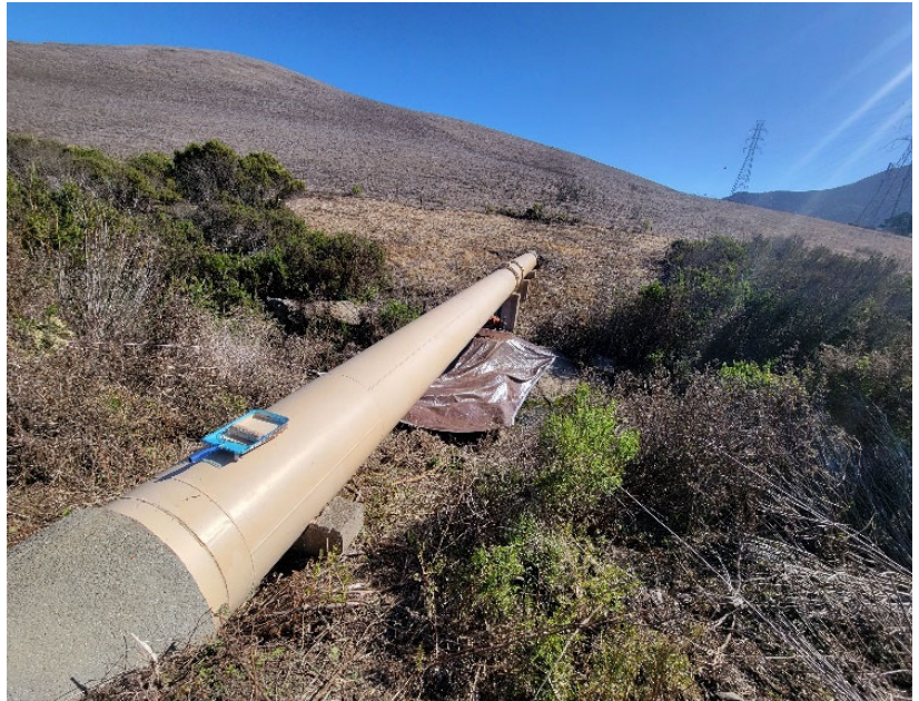
RECOATED PIPELINE CROSSING NEAR HWY 1
