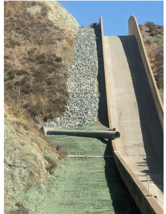
COMPLETED SPILLWAY UNDERDRAIN REPAIRS
