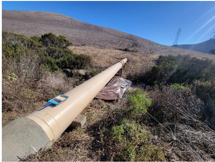
RECOATED PIPELINE CROSSING
