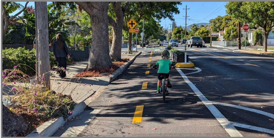
Protected Bike Lanes on Chorro Street Constructed with the North Chorro Greenway Project
