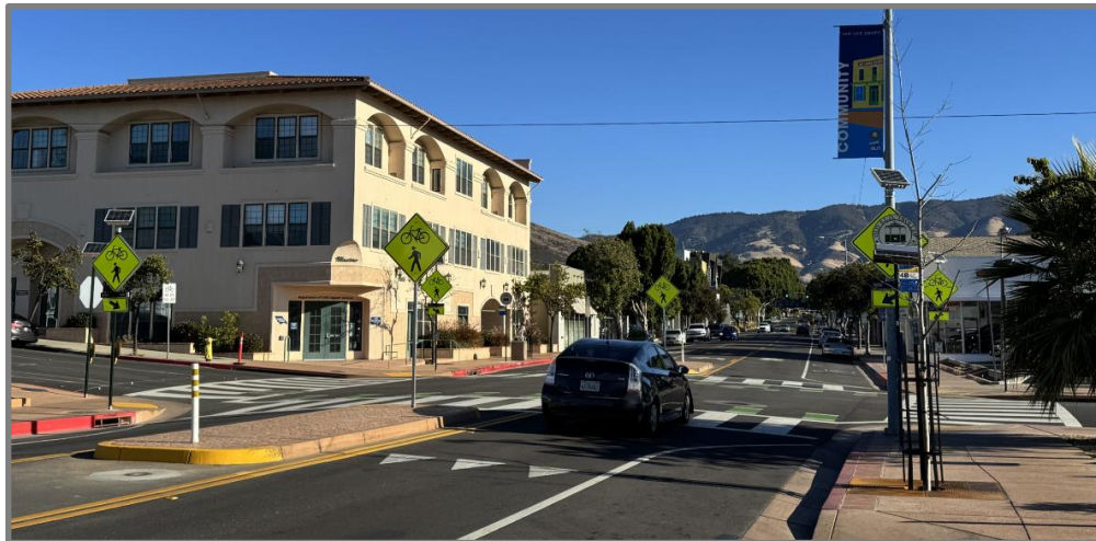
Enhanced Pedestrian Crossings on Monterey Street Installed with the 2023 Arterials Paving Project
