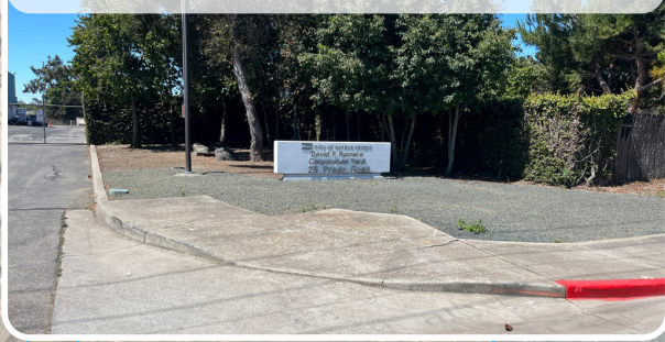
Existing City WRRF and Corporation Yard
