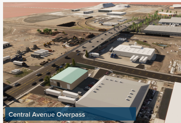
The Consor team recently designed a bridge in the City of Newark located in the San Francisco Bay Area that had many underground utilities. We slightly adjusted the locations of the bridge supports to avoid utility conflicts, reduce service impacts, and reduce project costs.
