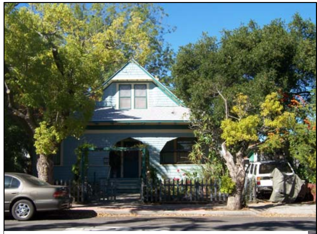
1344 Mill Street, South Elevation
