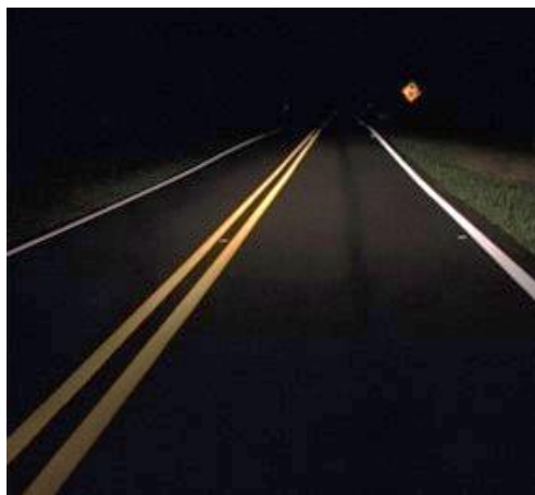
Example of Increased Nighttime Visibility with Addition of Edge Lines
