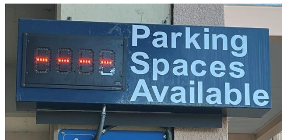
Figure 3. Existing Digital Occupancy Sign
