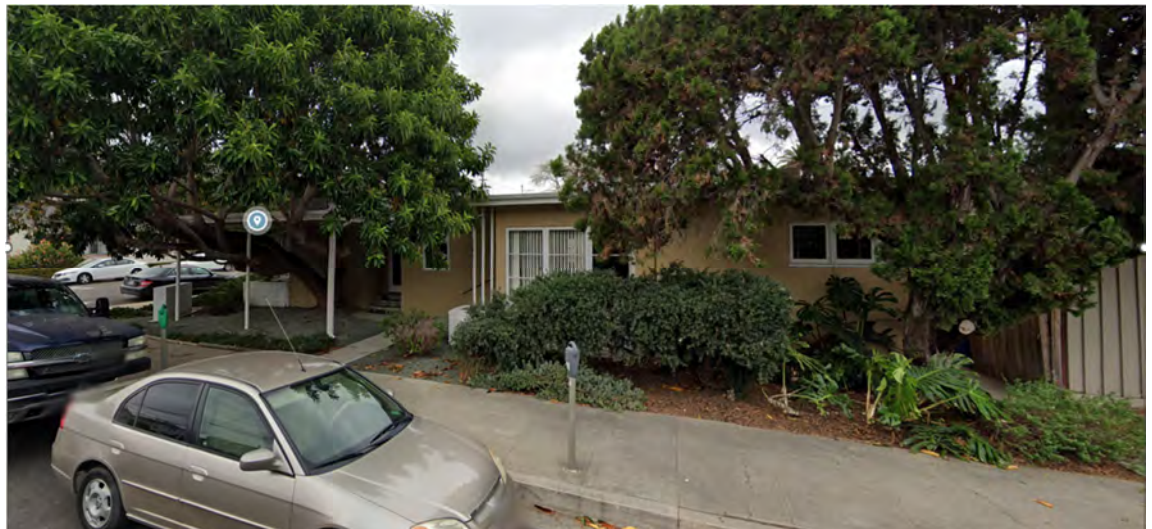
IMAGE 2 – PORTION OF BUILDING ON PISMO TO UNDERGO RENOVATIONS.
