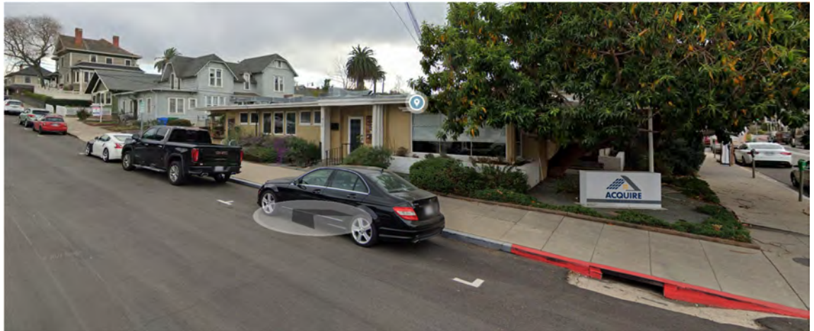
IMAGE 1 – PROMINENT CORNER VIEW OF EXISTING BUILDING
