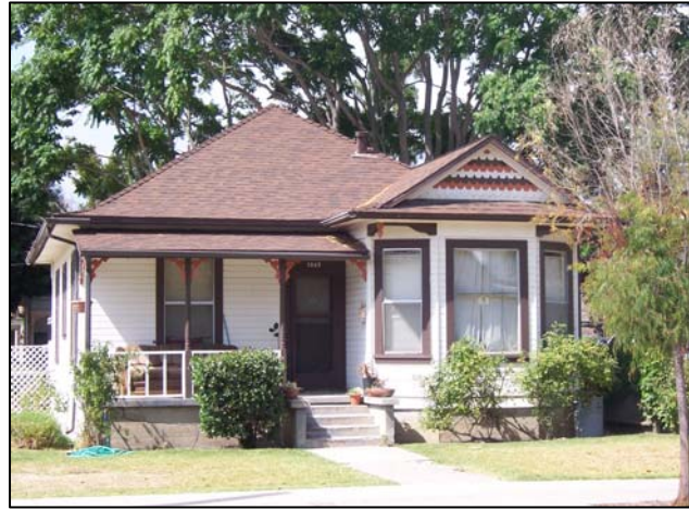
1543 Morro Street, East Elevation
