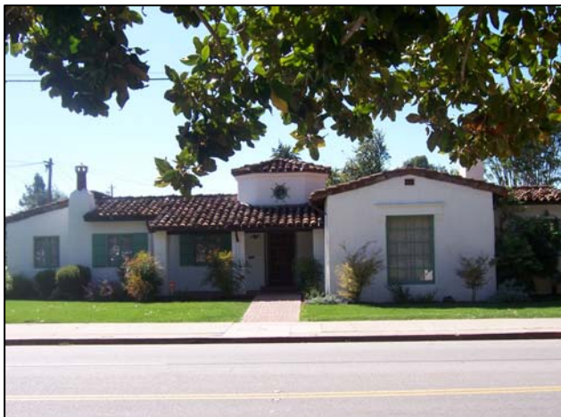
M.F. Avila House, 1443 Osos Street, East Elevation
