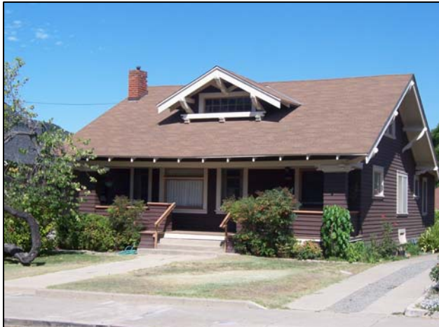
1060 Pismo Street, South Elevation
