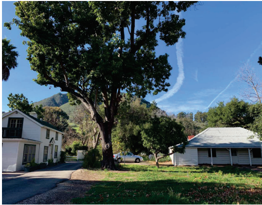
SOUTH SIDE YARD OF ADOBE
