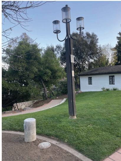
NOTE: REPLACE EXISTING POST LIGHT WITH NEW FIXTURE TYPE SP, PROVIDE GROUND ROD, AND 2-AMP FUSE IN ADVANCE OF LIGHT INSIDE EXISTING ROUND PULL BOX.
