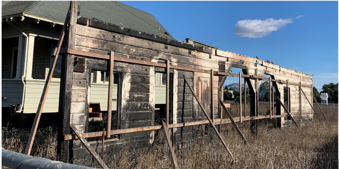
Figure 6: Fire-damaged Racetrack Grandstand Wall
