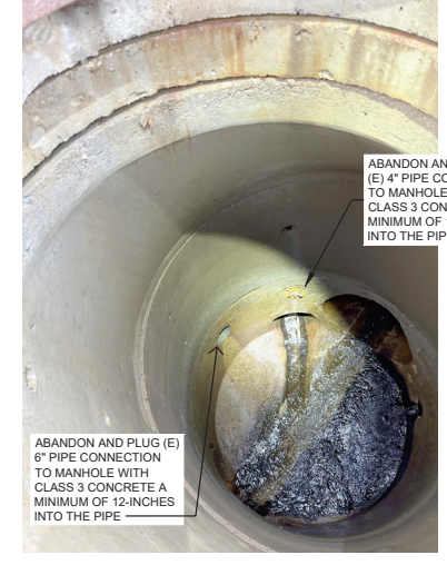
MH-11 DEMOLITION DETAIL NOT TO SCALE
