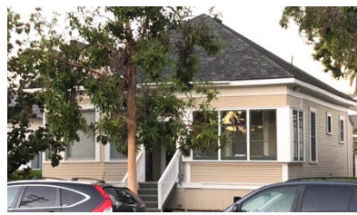
25. 1520 Morro (later porch enclosure)
