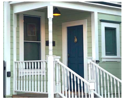
1533 Osos entry porch
