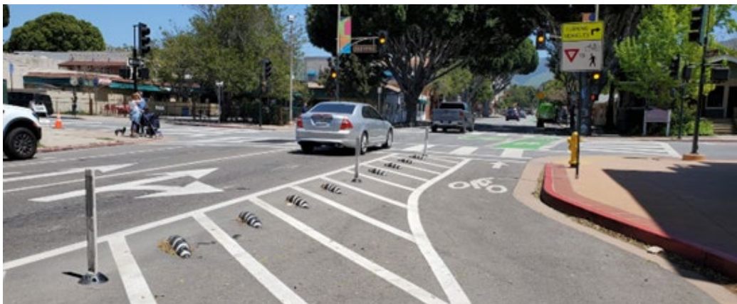
Example of Existing Mountable Protected Bikeway Separation on Marsh Street
