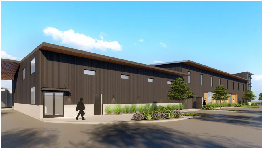
04 - VIEW FROM LOADING AREA
