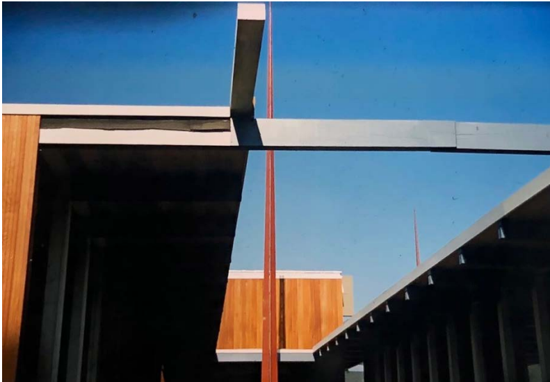
Mount Carmel, 1958, contrasting vertical church with horizontal annex. The flat roof, peaked at the truss, would later be replaced with a sloping roof, ancillary beam ends cut off, and both cedar siding and concrete base covered with stucco.
