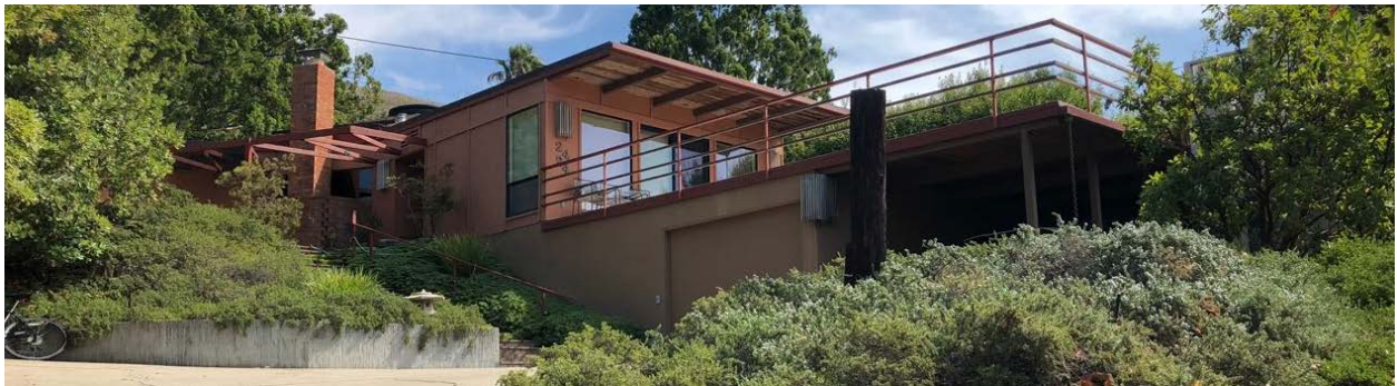
Page-Selkirk House from the street, showing stairs, living room spoke, and deck
