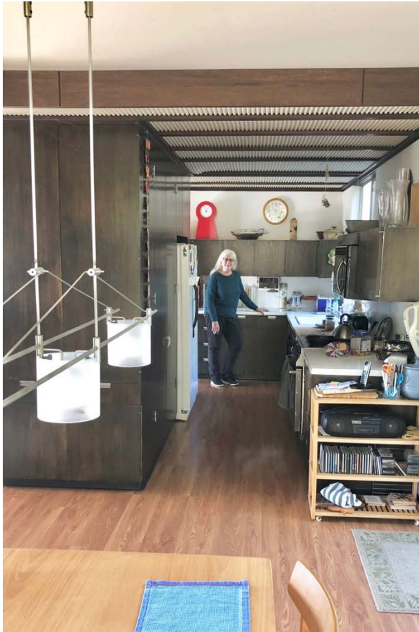
The dining room–kitchen axis with the kitchen’s full-length and -width, wood-framed, opaque plastic light panel
