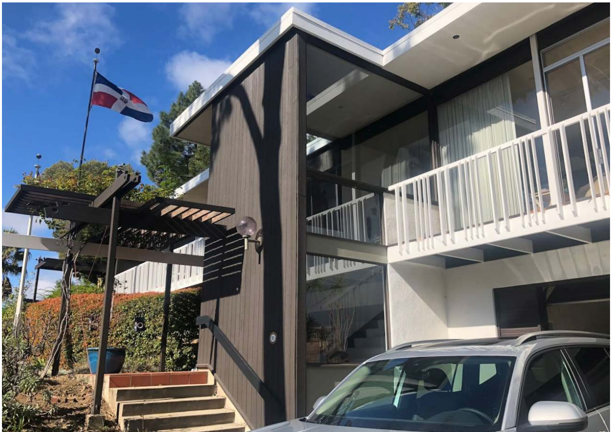
The stair tower entry to the Schwartz House: an inventive adaptation to the site that subtly but dramatically communicated a sense of arrival to generations of activists and politicians.
