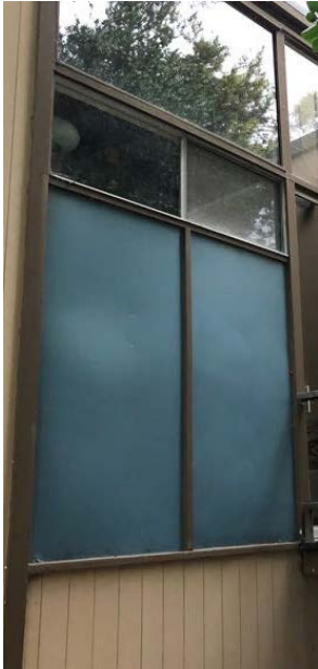
Pimentel-Orth House: Fixed glass, sliding window, Masonite, V-groove shiplap
