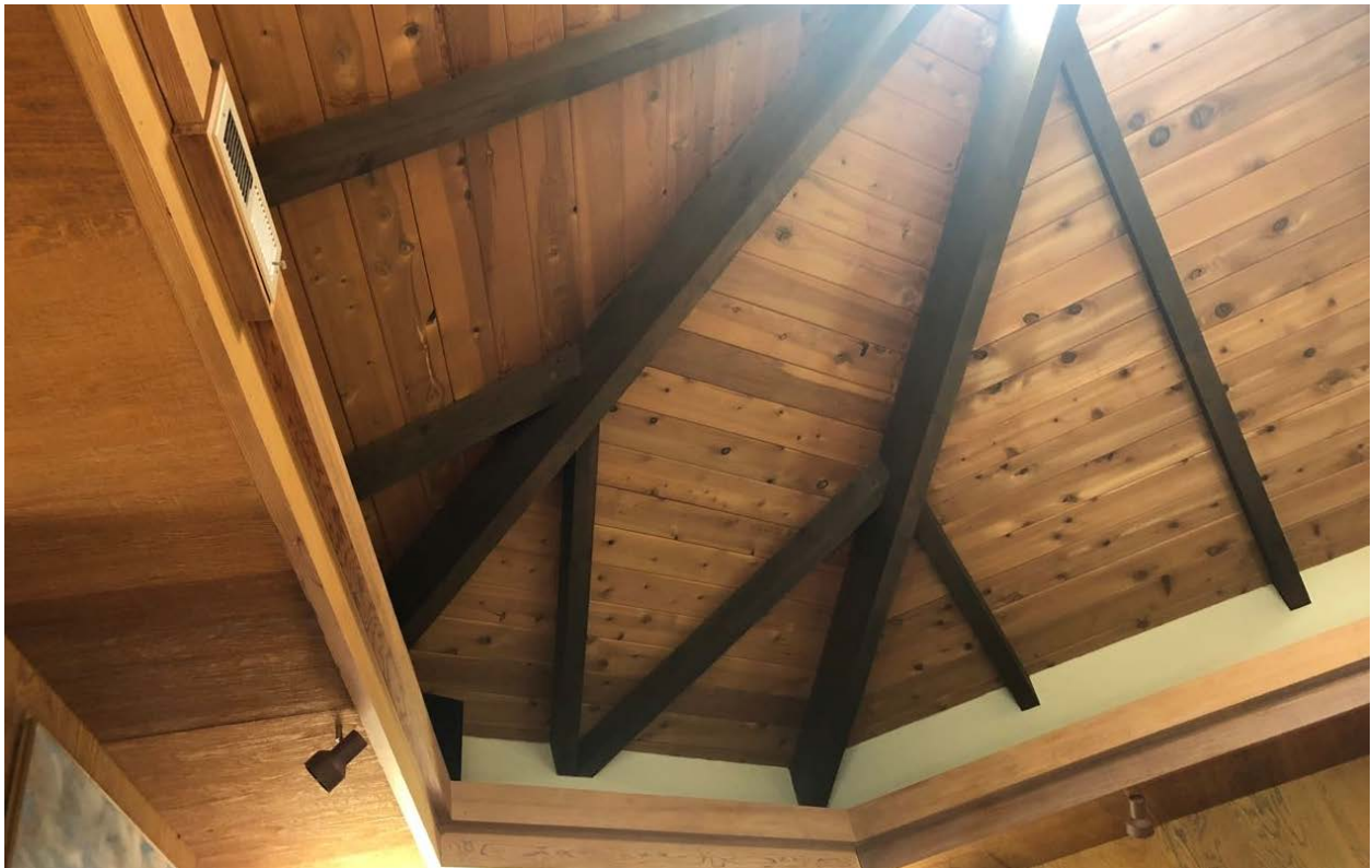
Redwood plywood walls and soffits rise to a complex network of rafters with a plank ceiling and hexagonal skylight in the Page-Selkirk house.
