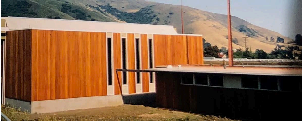
Mount Carmel, 1958, contrasting vertical church with horizontal annex. The flat roof, peaked at the truss, would later be replaced with a sloping roof, ancillary beam ends cut off, and both cedar siding and concrete base covered with stucco.
