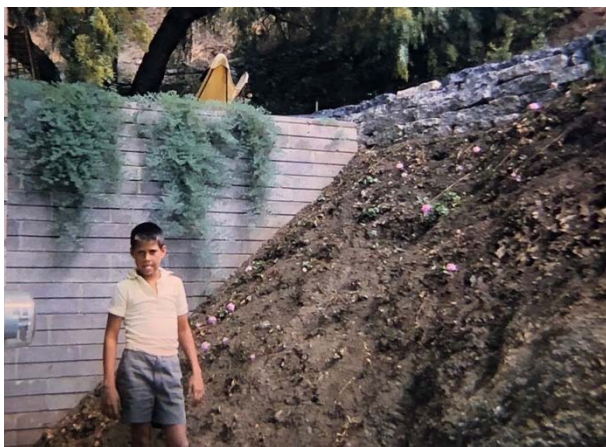
Jan with one of his retaining walls
