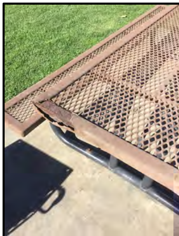
Figure 15b. Picnic Table with exposed metal
