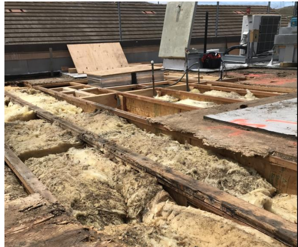
Photo #2 – Rotted Structural Members
