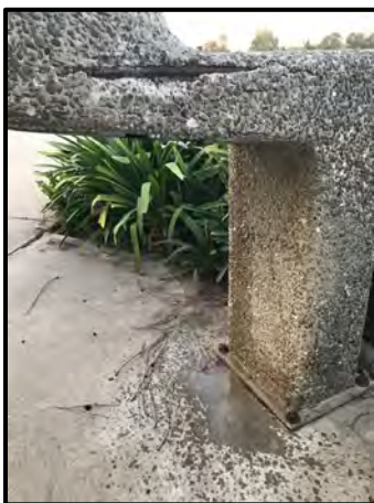
Figure 14b. Leaking cement drinking fountain
