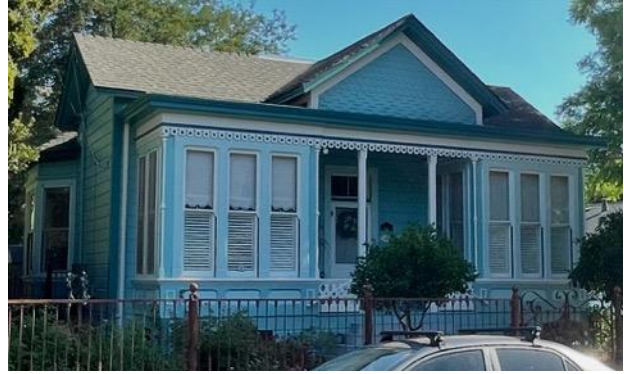
Dana-Barneberg House now, absent ridge cresting and gable finial
