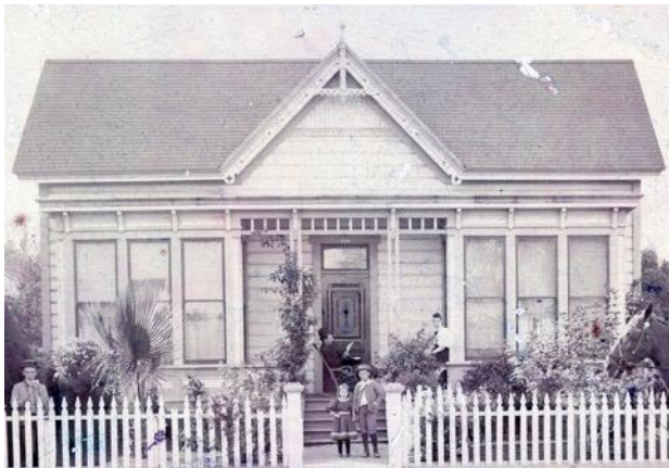
McCabe House in original form
