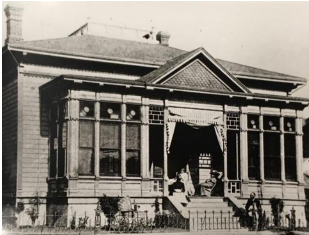
Goldtree House as an Italianate cottage with double-bay Eastlake porch attached
