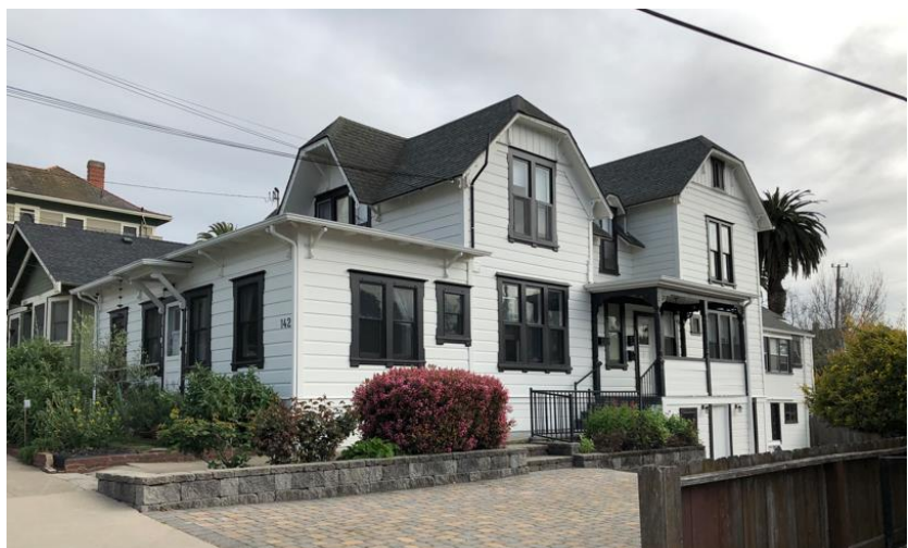
Figure 1: Meredith House (1421 Garden St)
