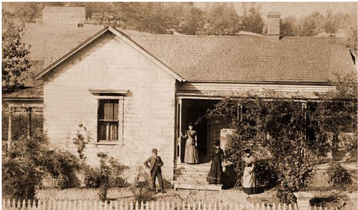
The Guthrie-Bianchi House's pierced columns around the turn of the century, with spindle columns on the porch at far left.
