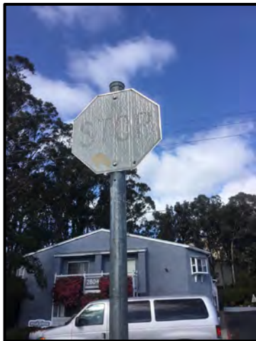
Figure 13a. Faded Stop sign
