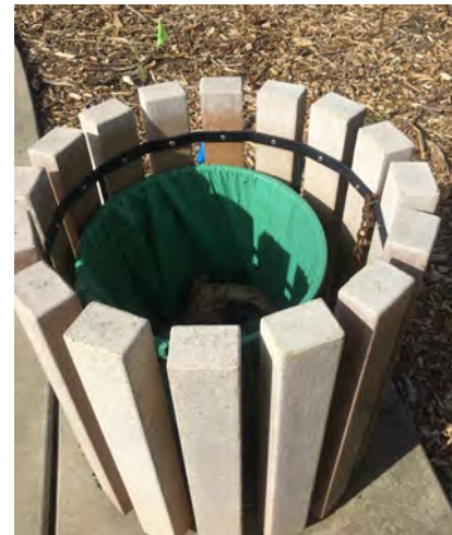
Figure 21a. Incorrectly sized trash bin
