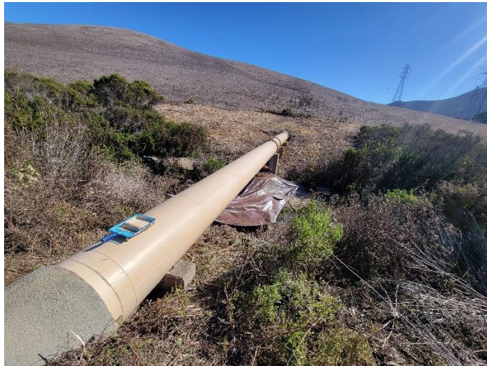
RECOATED PIPELINE CROSSING
