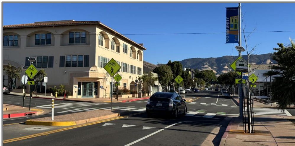
Enhanced Pedestrian Crossings on Monterey Street Installed with the 2023 Arterials Paving Project
