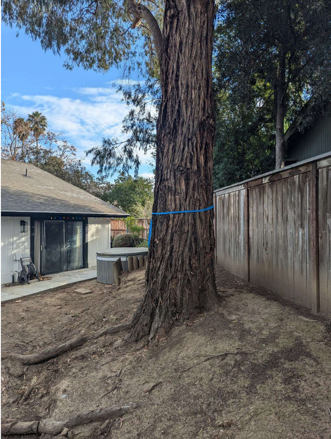
Side view of trees on 2:1 slope. Note proximity to fence and adjacent residential houses.
