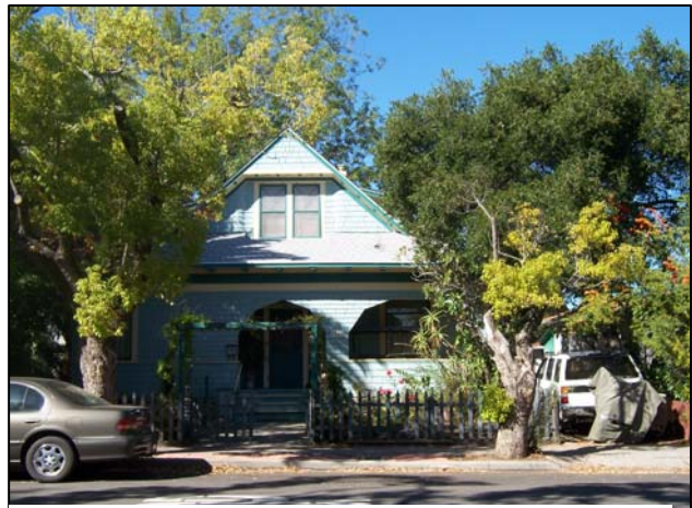
1344 Mill Street, South Elevation
