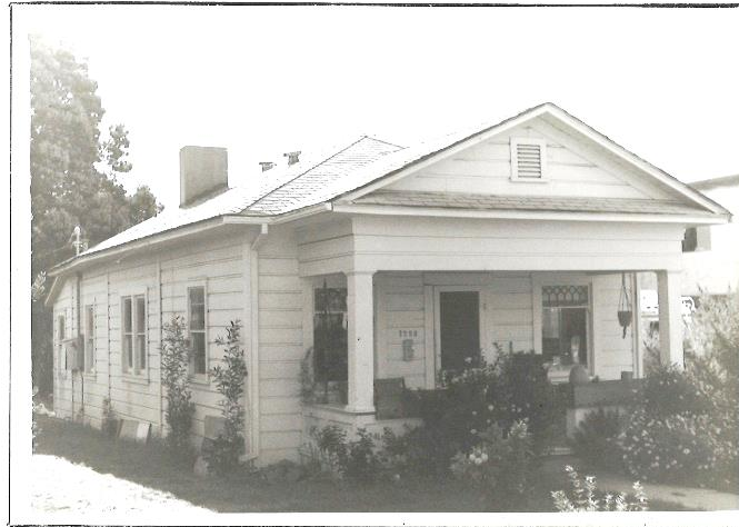
1253 Mill: This Neo-Classical rowhouse has a hipped roof with a centered gable porch with square columns supporting a plain pediment. Diagonal latticed windows accent the residence.
