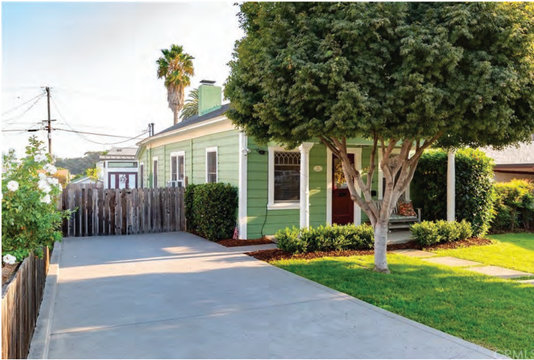
VIEW DOWN DRIVEWAY EXISTING
