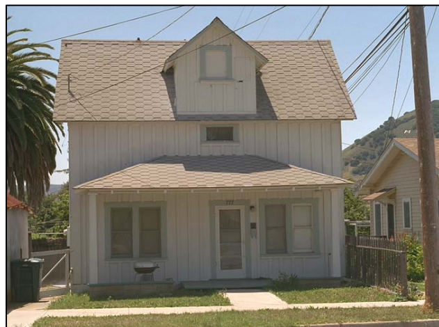
777 Johnson Avenue, East Elevation
