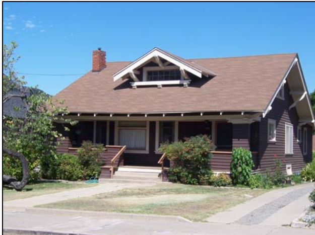
1060 Pismo Street, South Elevation
