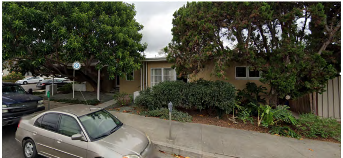
IMAGE 2 – PORTION OF BUILDING ON PISMO TO UNDERGO RENOVATIONS.
