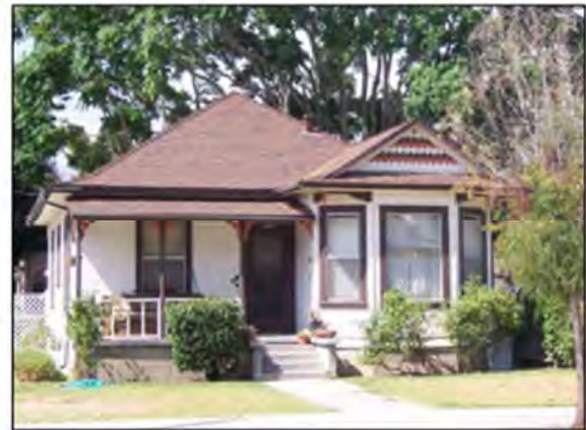
1543 Morro Street, East Elevation
