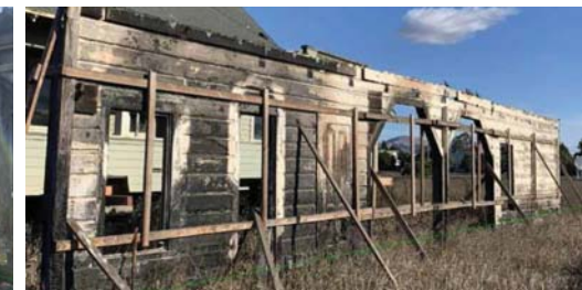
REUSE OF EXISTING "BURNT WALL" FACADE OF VIEWING BARN FOR INTERPRETIVE DISPLAY.
