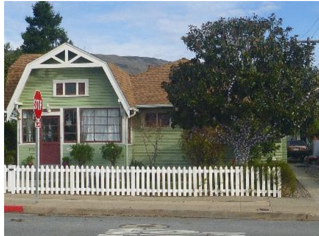
Figure 4: Bittick Residence, 1902 Chorro
