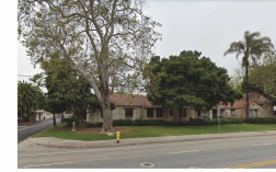
3 1-STORY BUSINESS NORTH OF THE SITE
