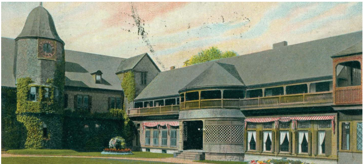
Bellcast roof of tower (left) and curved porches (center) of the Newport Casino
