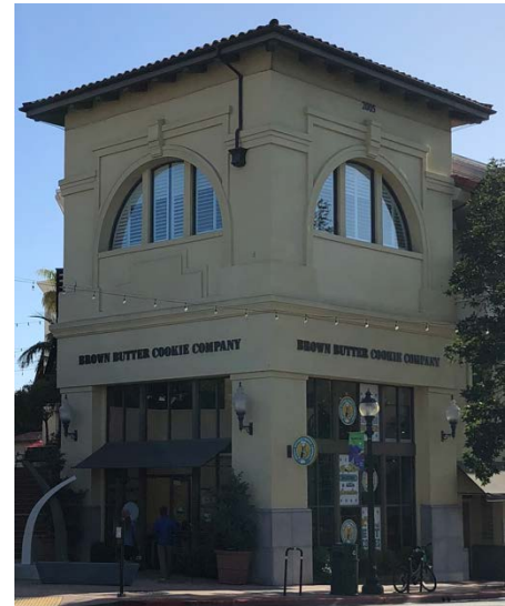
Below: Diocletian windows with faux keystones crowning Court Street Shopping Plaza
