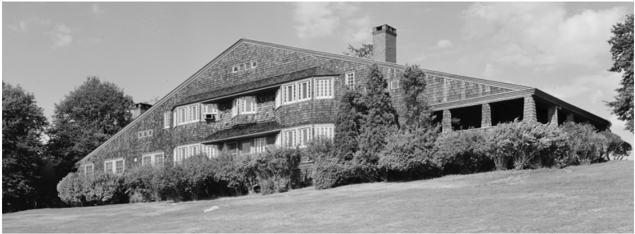
William G. Low House, McKim, Mead and White, 1885–1887: in the form of a single encompassing gable. HABS photograph before demolition.
