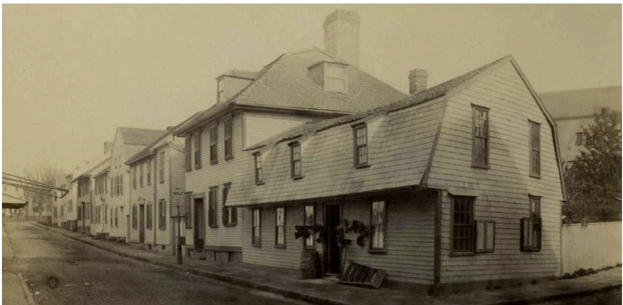
Hip, front- and side gable, and gambrel roofs on clapboard and shingle houses in one of Stillman's 1874 Newport photographs, entitled "Tory Corner Thames Street" in McKim's handwriting. Newport Historical Society.
