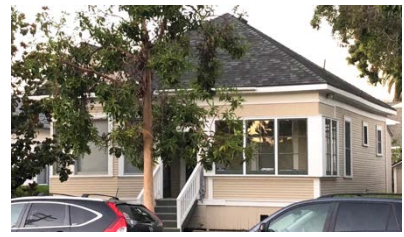
25. 1520 Morro (later porch enclosure)
