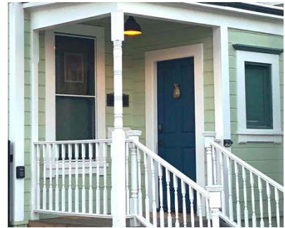
1533 Osos entry porch
